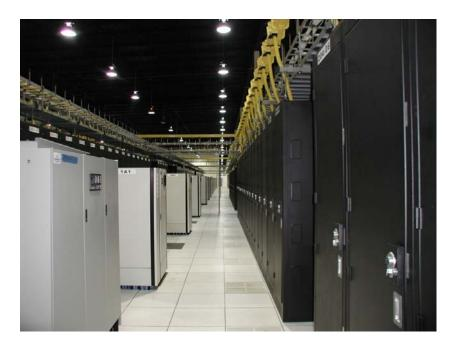
Figure 4. Rows of UPS fed Power Distributing Units (gray cabinets) feeding power to rows of IT equipment (Black cabinets)
