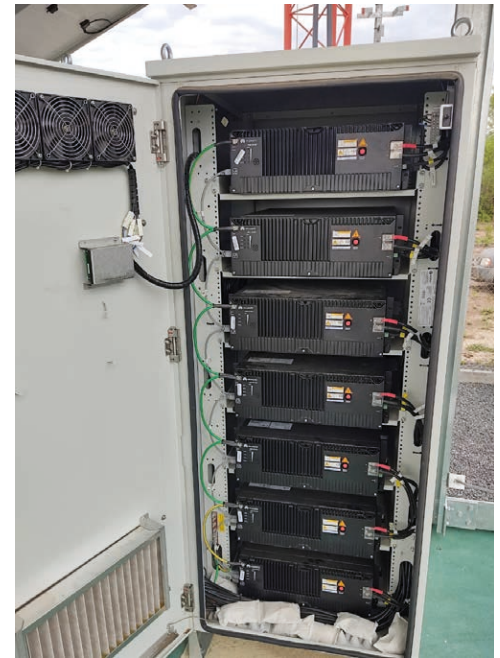
Vertiv™ EPC 48300/2900 outdoor cabinet with lithium-ion batteries
